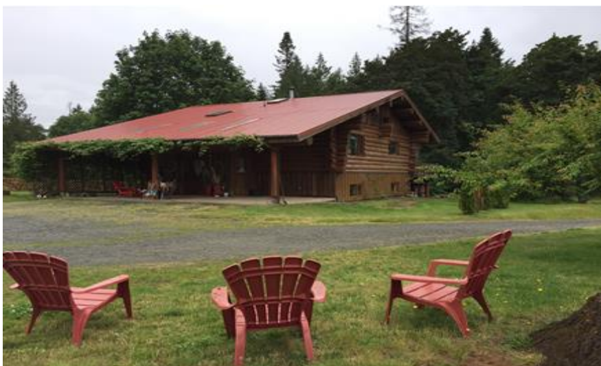
Figure 2: Existing Single Family Dwelling (to be retained on proposed Strata Lot 1)
