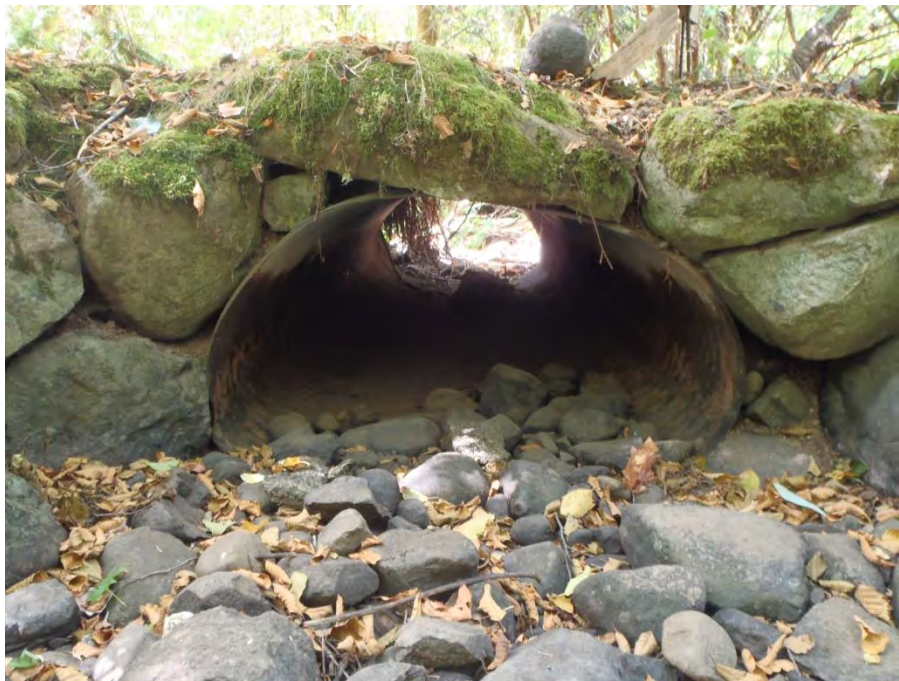
Photo 6. View upstream of the existing Tributary 11 crossing that will be upgraded during Copperfield Road ROW development. (Aug. 30, 2017).
