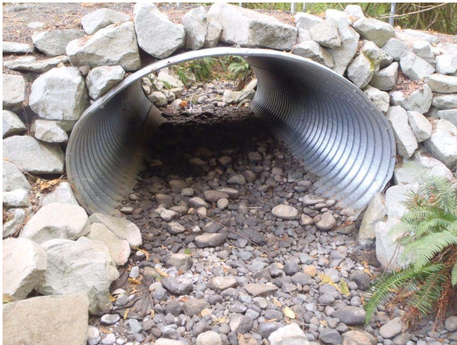
Photo 5. View upstream of the existing pedestrian trail culvert crossing across Piercy Creek mainstem located near the southern property boundary. (Aug. 30, 2017).
