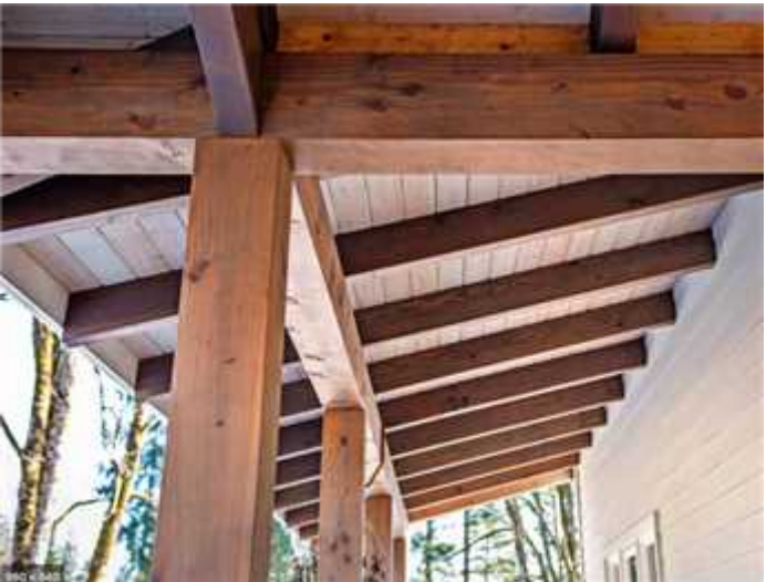
D-FIR , TIMBER FRAME DETAILS STAINED
