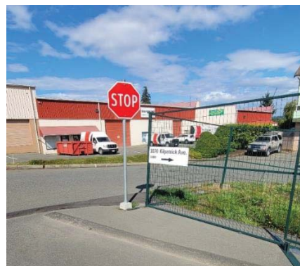
10. Another view of the internal stop sign as it exists at the intersection of the parking lot on the prosed site and the north driveway. Drivers run through it consistently. It could benefit significantly from the addition of a white stop line.
