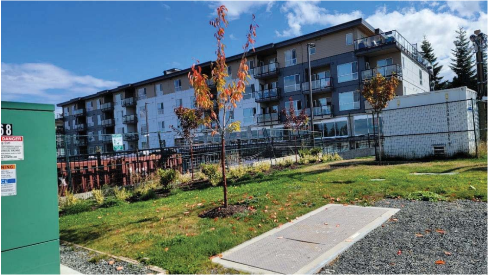
2. View of the commercial spaces in building 2 of Newport Village from the sidewalk. Imagine a 5-story residential block the entire width of the undeveloped lot behind this construction fence. Then imagine a small commercial space on the northwest corner and the portion of the site visible here as parking spaces, bringing commercial traffic into direct view of the commercial spaces in building 2.
