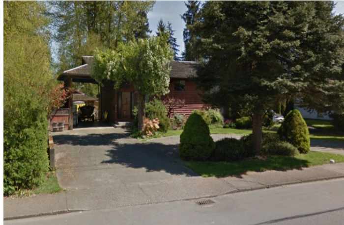
Figure 2: View of subject property from Willemar Avenue
