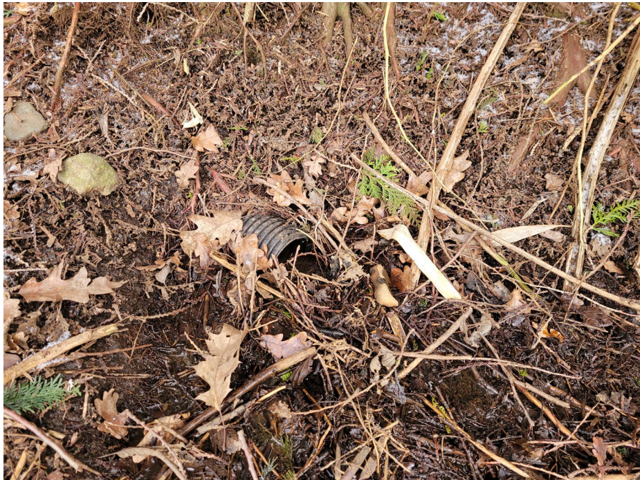
Photo 22. Pipe beneath residential property contributing flow to Ditch 1 (February 2021).
