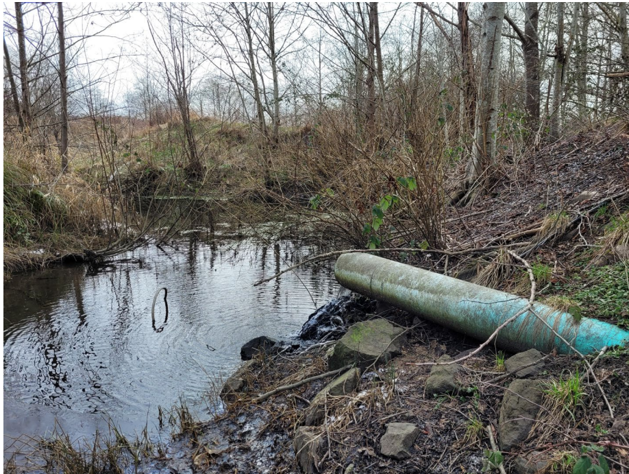
Photo 14. Pipe in the northwest corner of Len's pond that diverts overflow water from the culvert beneath 801 Ryan Road into the pond (February 2021).
